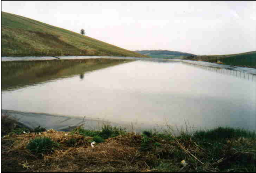
Picture 5. Large lagoon for storing digested pig slurry
